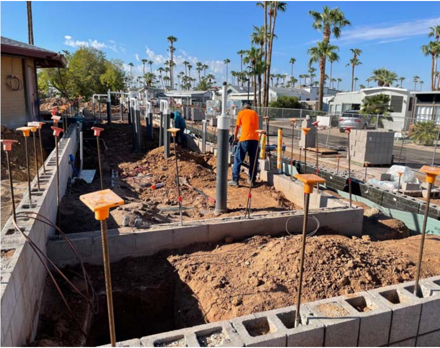
Pump house for west
