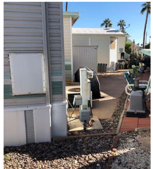
NON-COMPLIANT LIVABLE STRUCTURE
